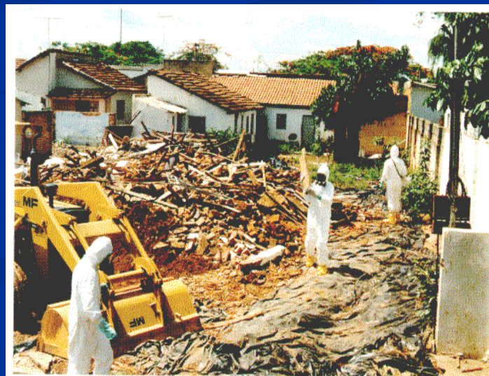
13. Contaminated rubble from the demolition of R.A.'s house on 57th Street.
